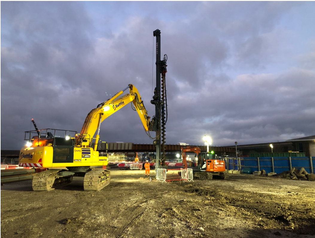
Figure 1: Our Komatsu PC490 with Movax attachment completing some sheet piling
